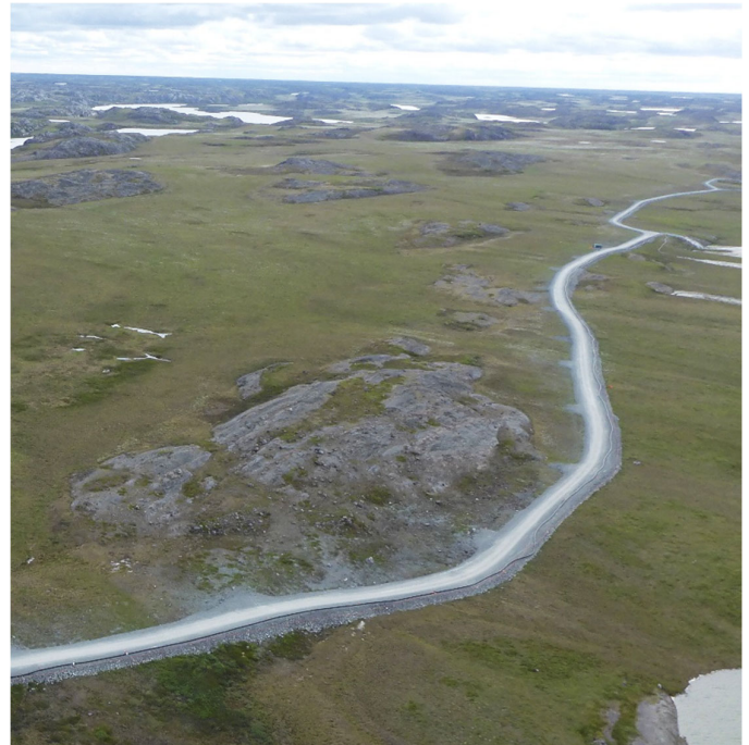
Run-of-quarry rock road embankment constructed on ice-rich permafrost soils in Nunavut, Canada
