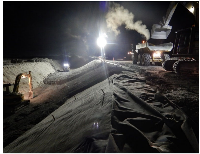
Winter excavation of a key trench during construction of a frozen foundation tailings dam in Nunavut, Canada
